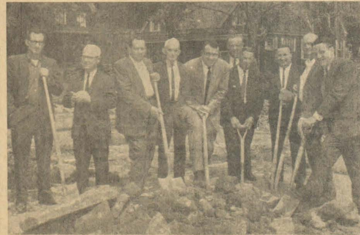
Excavation work preliminary to construction of the Floyd county courthouse on a new site here was begun Monday morning by Akers & Akers, contractors. Shown here at the groundbreaking are, from left: Magistrate Edward Caudill, Burl Spurlock, president of the First National Bank, County Judge Henry Stumbo, Trial Commissioner Glenn C. Burchett, County Attorney Barkley J. Sturgill, Jailer Lawrence Hale, Magistrate Fred Conn, County Clerk C. Ollie Robinson, Magistrate Zeb Ousley, H. D. Fitzpatrick, Jr., vice-president of The Bank Josephine.
