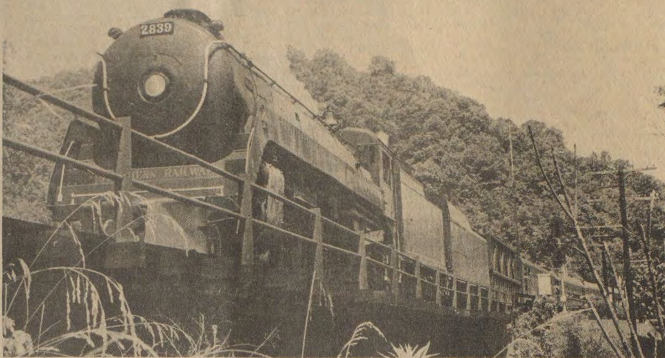
WITH A PUFF, A HISS, AND A CLANG, a steam locomotive draws away from West Prestonsburg station last week, on its way to Elkhorn City, the next leg on its journey from Lexington to Spartanburg, South Carolina. The train carried passengers on an excursion organized by the Blue Grass Railroad Club of Lexington.
